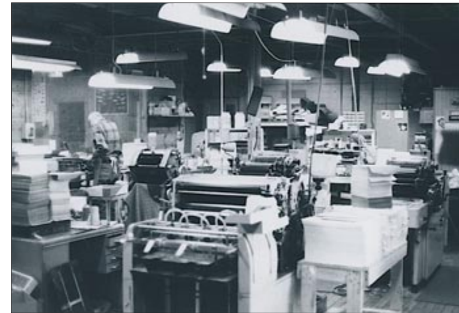
Commercial Street pressroom
