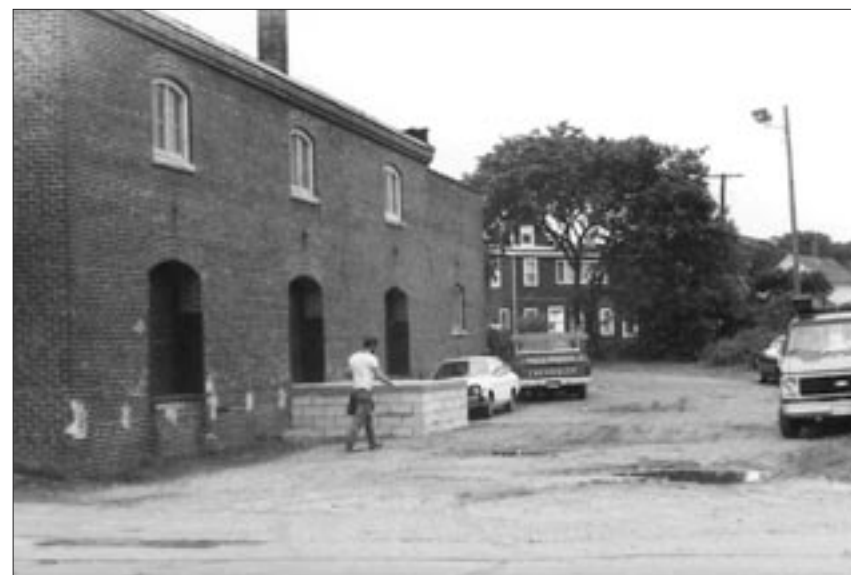
Building the loading dock at Maplewood Avenue
